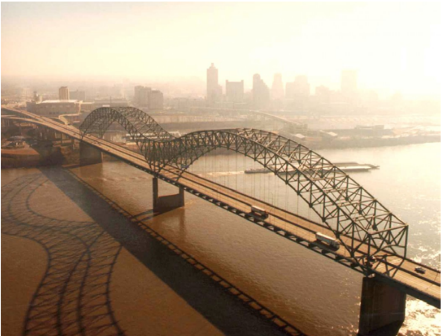
Aerial view of the Hernando de Soto Bridge across the Mississippi River between Memphis, Tennessee and West Memphis, Arkansas, USA. The bridge was opened in 1973 and carries six lanes of Interstate 40 across the river. View is from the Arkansas side to the east-southeast across the river to Memphis. Photographer Larry Donald, U.S. Army Corps of Engineers.
