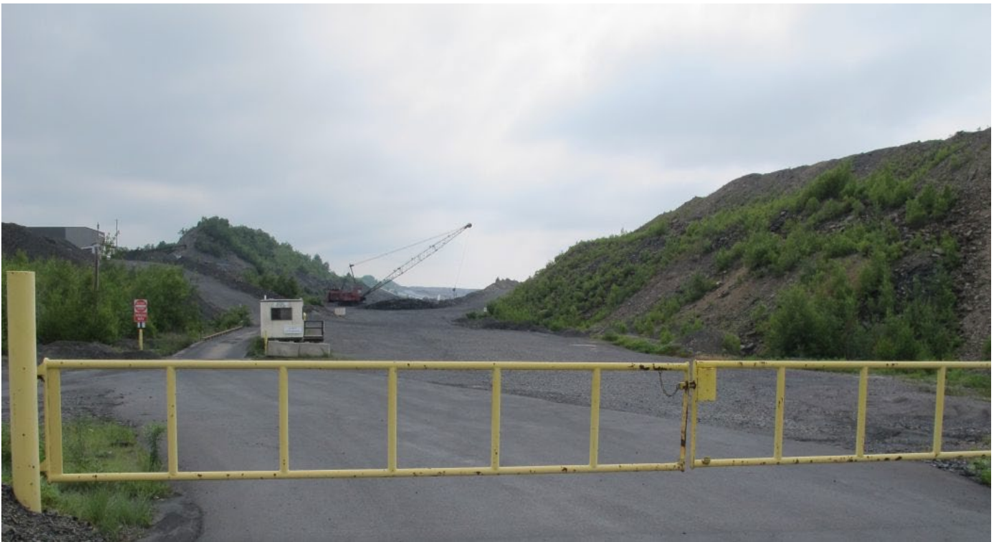
Mining near Stockton, PA, showing the culm banks on both sides of the road. Image by Paul Shackel, 2012.
