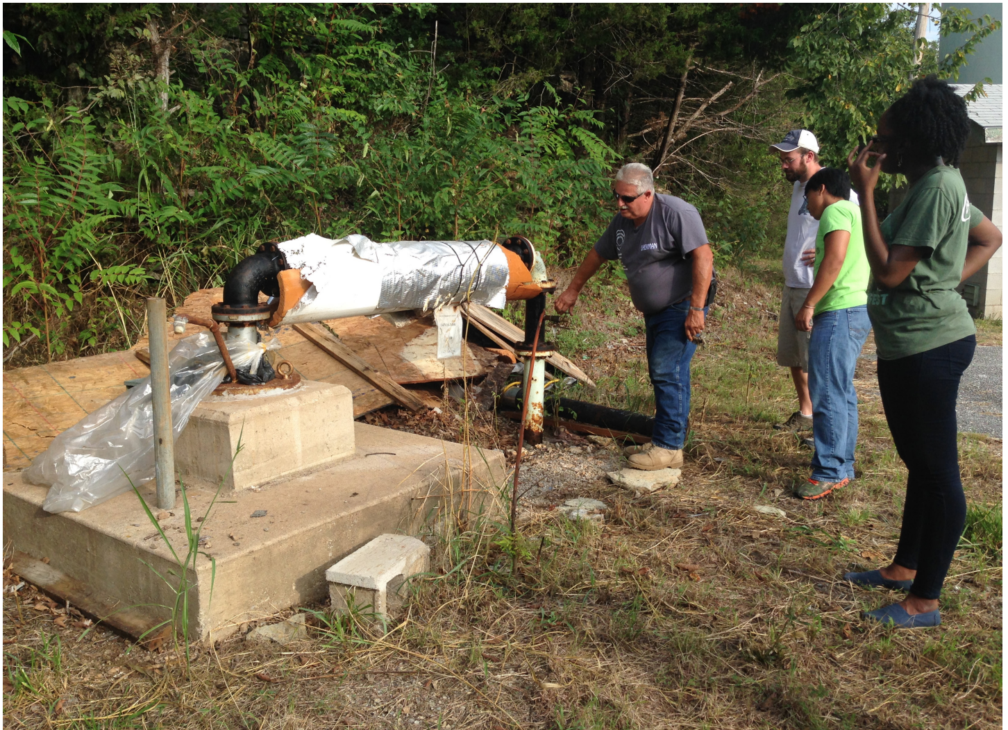
Learning about the condition of water infrastructure in Sulpher Springs, Arkansas, for Water Bar at Crystal Bridges Museum.
