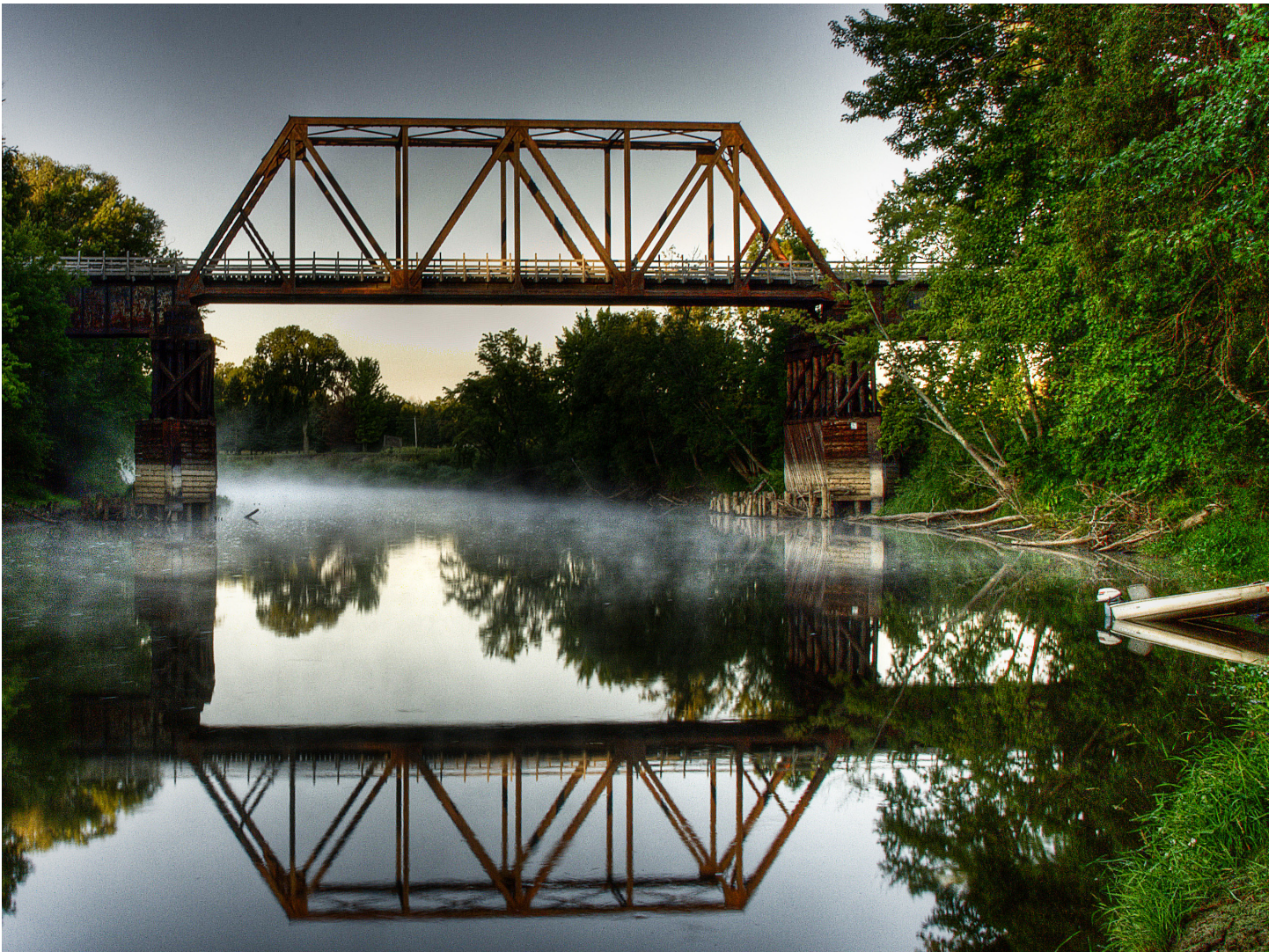
Steel truss bridge over the Mississippi River in Palisade, MN. Image courtesy of Peter Ladd, 2009.
