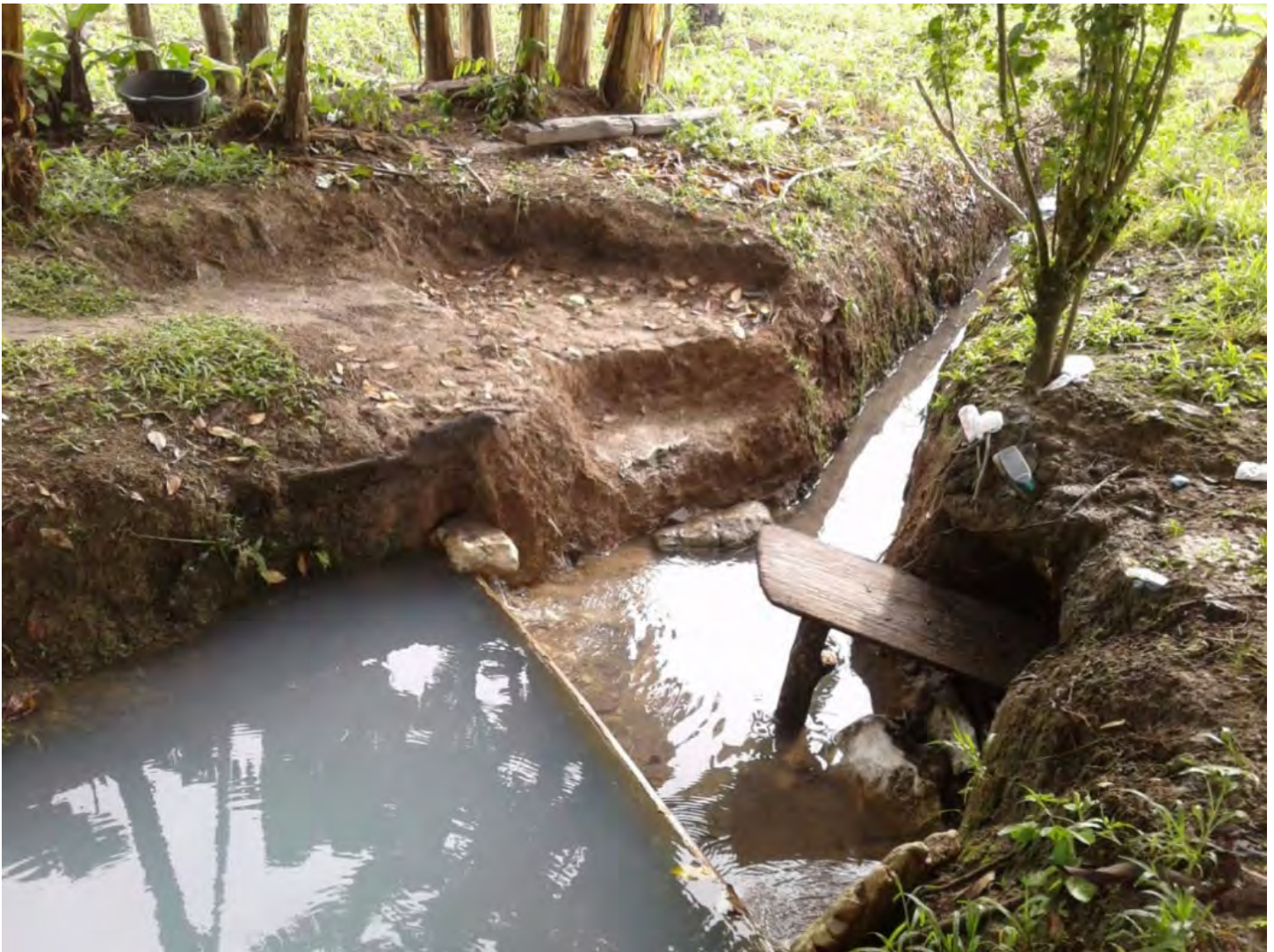
Figure 5. Reuse of ancient depressions or wells with a trench dug connecting the two wells and evidence of a filtration system set up. Image courtesy of William G. B. Odum.
