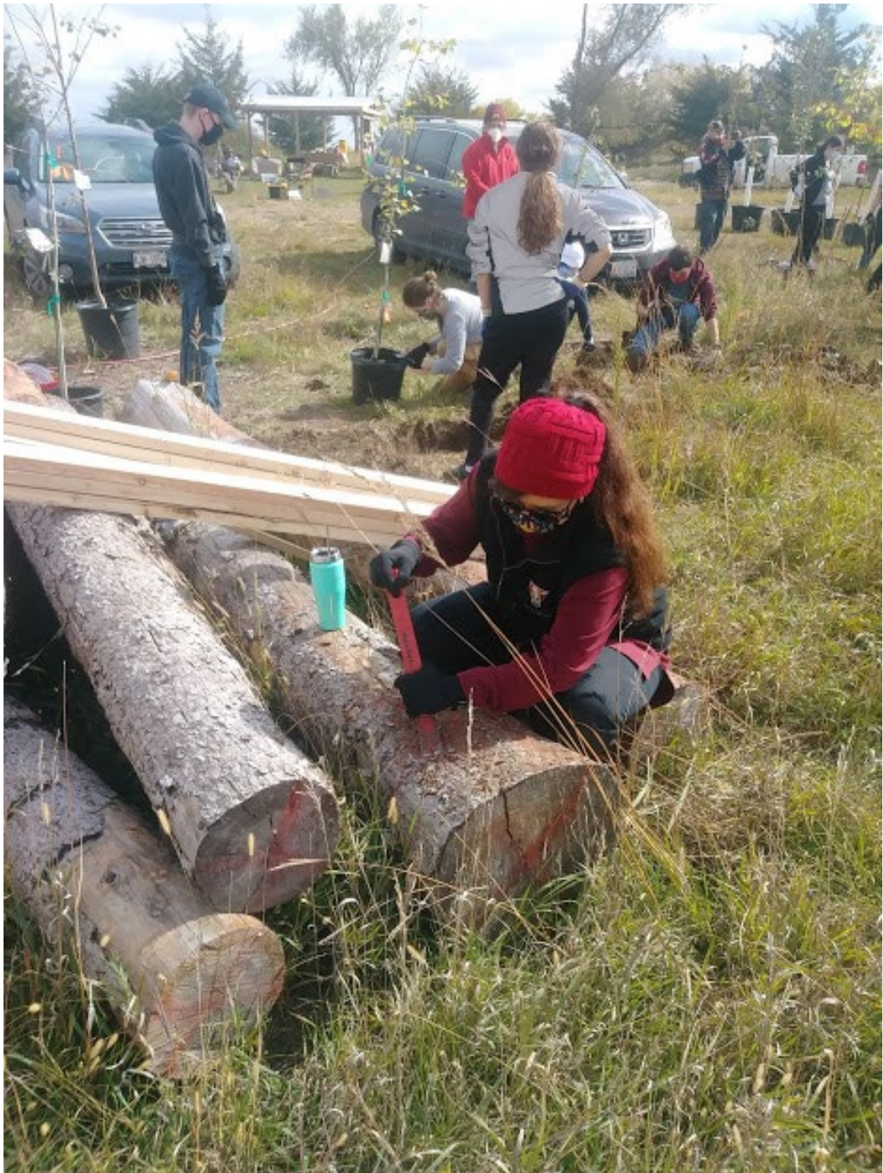
Many hands make light work at Zani Otunwe. Governing council member Roxanne Biidabinokwe Gould is shown here stripping bark from the many logs used in earthlodge building. Image courtesy of Waziyatawin.
