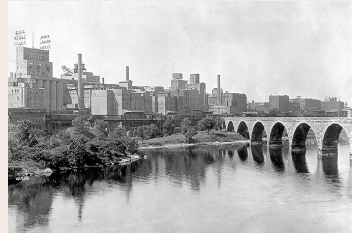
Stone Arch Bridge, 1960
