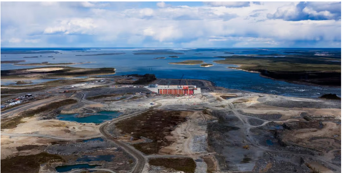
Detail from The Keeyask Dam site on the Nelson River, 2019. Image courtesy of Aaron Vincent Elkaim.
