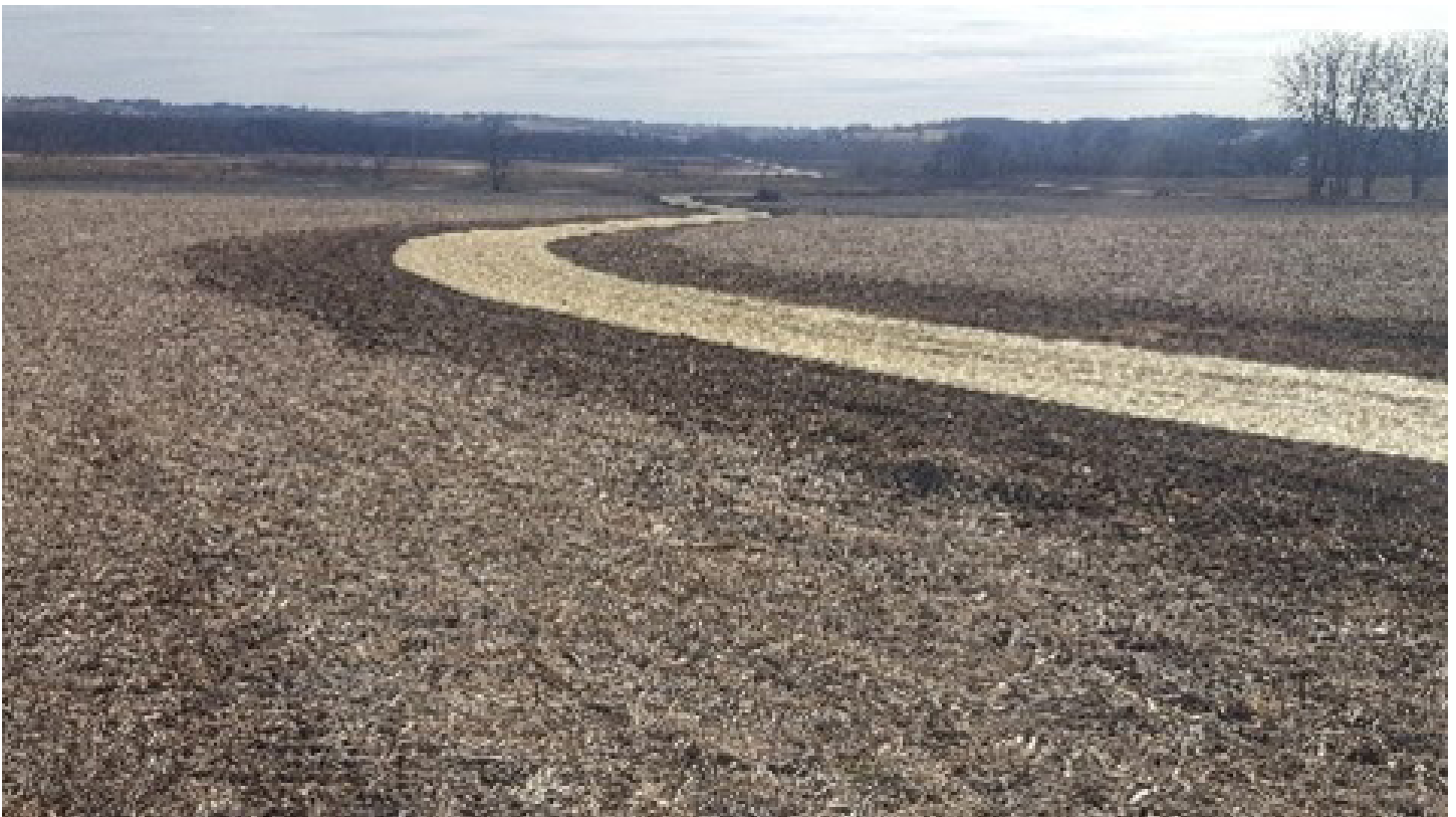
These waterways are purposefully shaped and planted with strong-rooted grasses to help channel water above ground and off the farm after weather events. The lighter area in the photo has been shaped and planted with grass seed in a straw mat to help with establishing the grasses. Image courtesy of Mollie Aronowitz.
