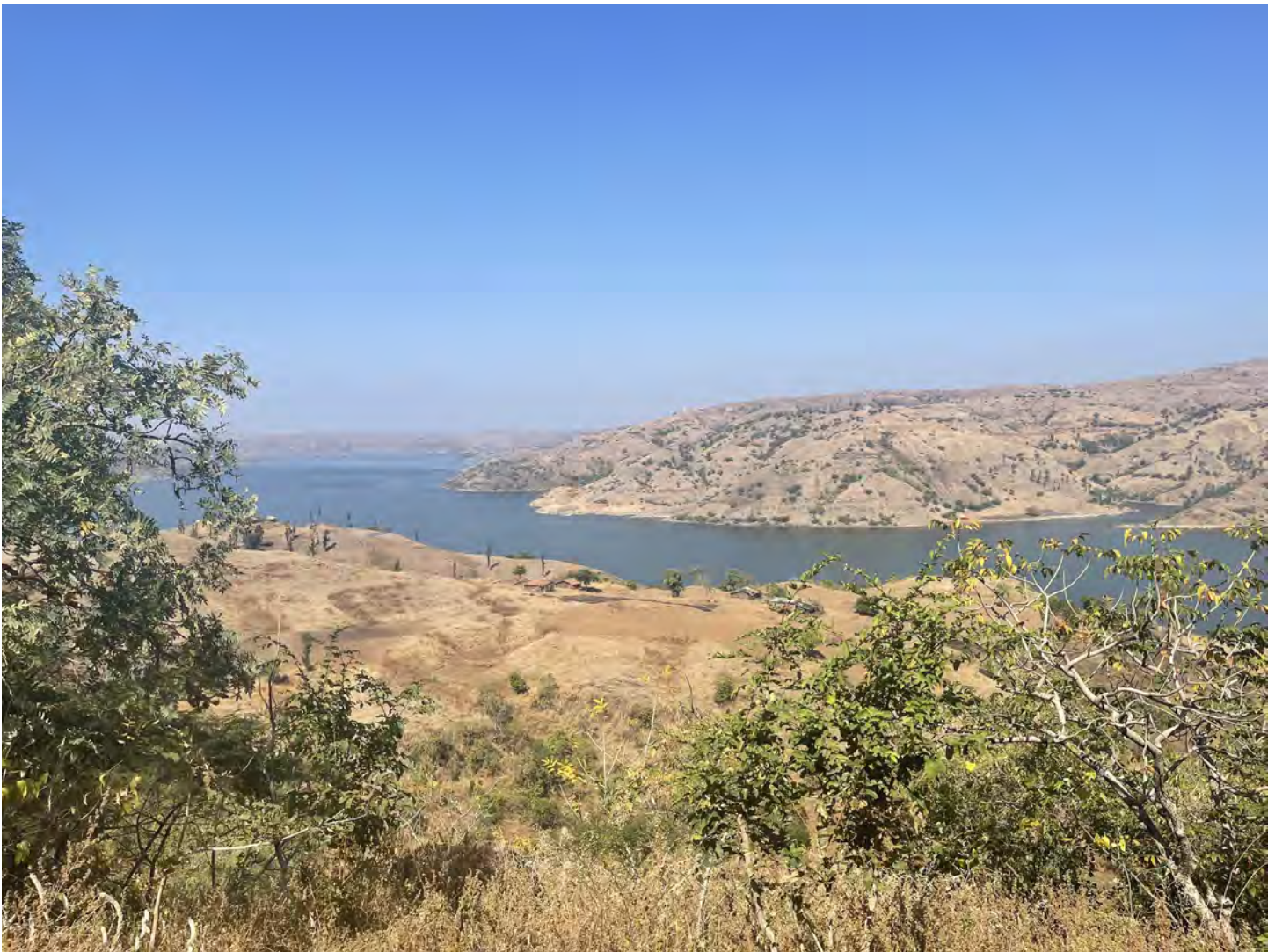
The deforestation is apparent here at the boundary of Madhya Pradesh and Maharashtra, where the Sardar Sarovar Dam's reservoir extends over two hundred kilometers upstream. Image courtesy of Vivek Ji.
