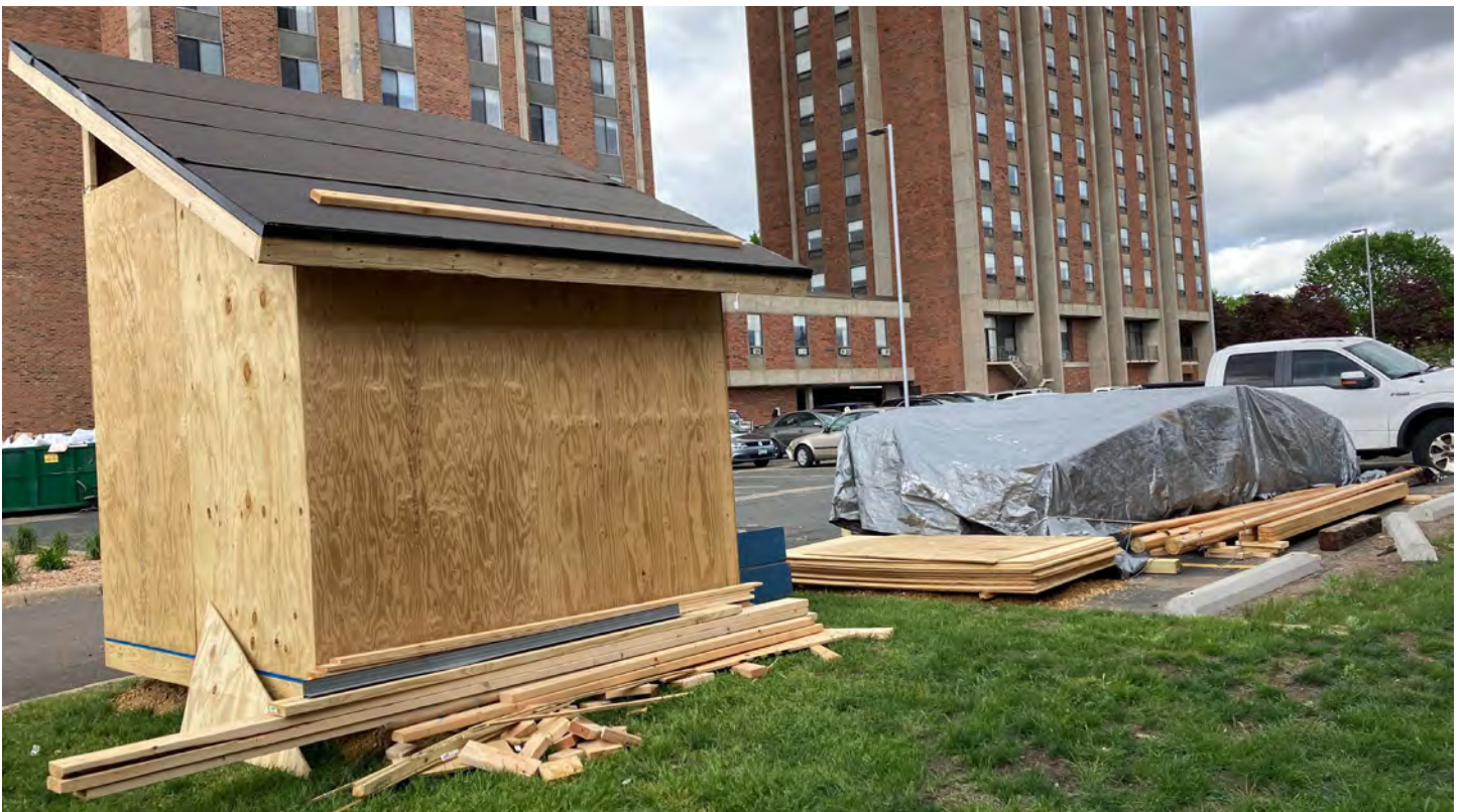
The solar shed, now framed and covered with tar paper on the roof, sits on the edge of a parking lot at Augsburg University. Image courtesy of Joseph Underhill.
