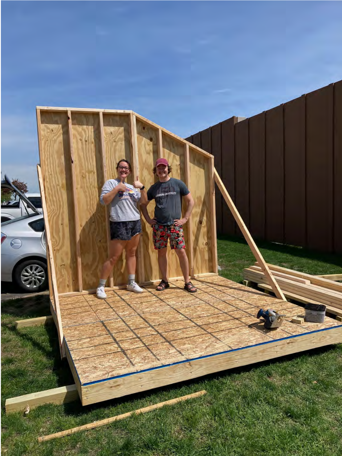
The floor and one wall of the solar shed as it is being framed. The shed sits on two four-by-four wooden beams. Image courtesy of Joseph Underhill.
