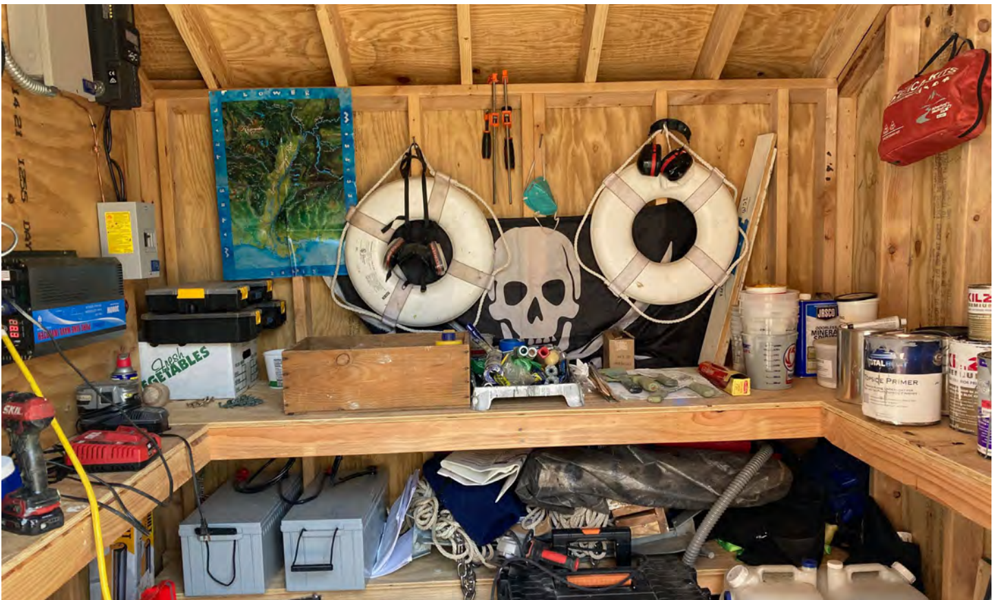
The shed's interior shows two batteries (grey boxes on the lower left), a charger and inverter (on the wall on the upper left), and various tools, flags, and supplies. Image courtesy of Joseph Underhill.
