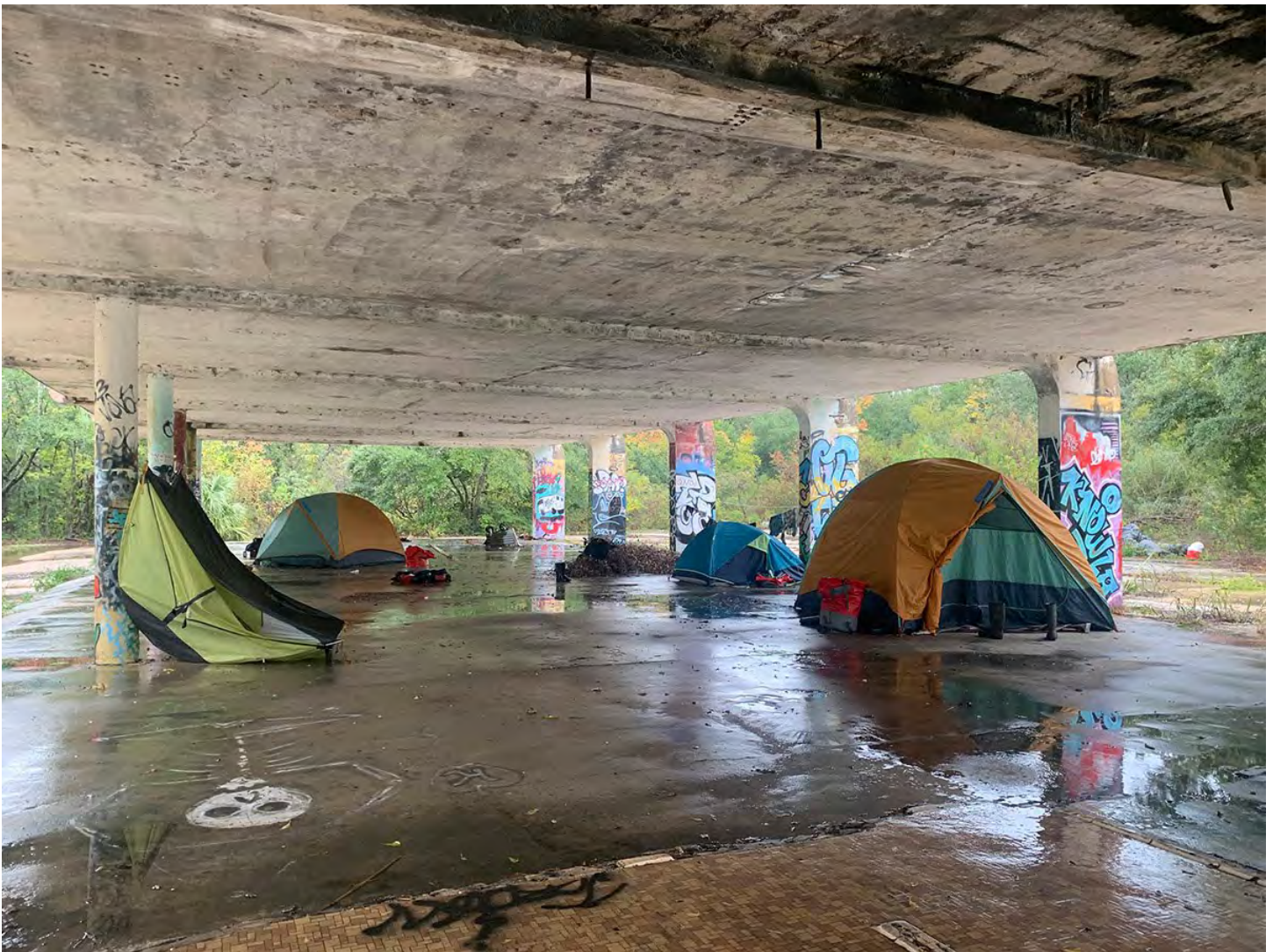
Tents set up under an abandoned structure at Lincoln Beach, Louisiana, during a rainy day. Image courtesy of Stephanie Lindquist.
