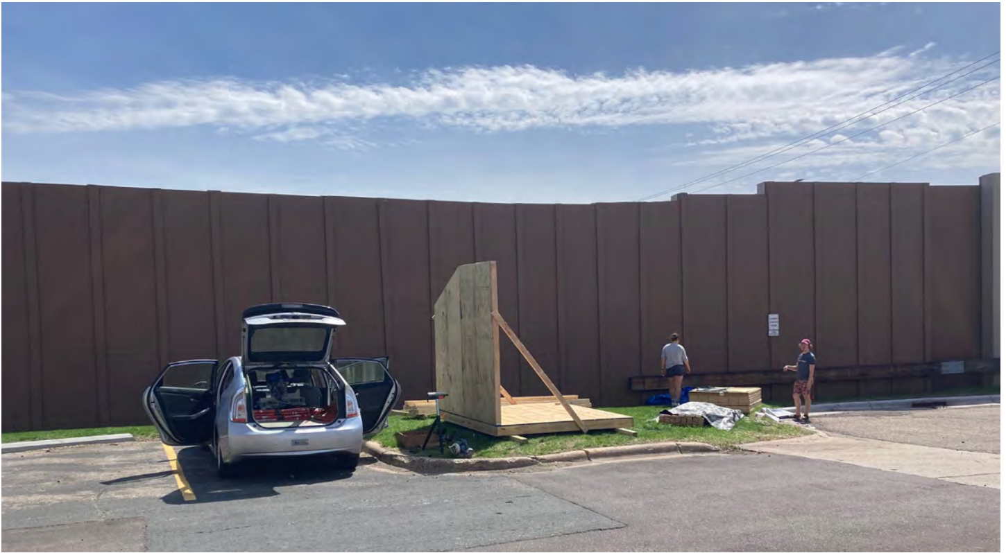
The solar shed is located on the edge of a parking lot on the Augsburg campus by the I-94 freeway wall. Image courtesy of Joseph Underhill.
